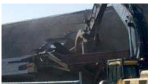
Photo Gallery: Manchester Parkade 'Dark Side' Demolition
