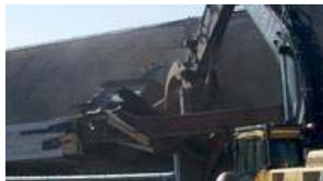
Photo Gallery: Manchester Parkade 'Dark Side' Demolition
