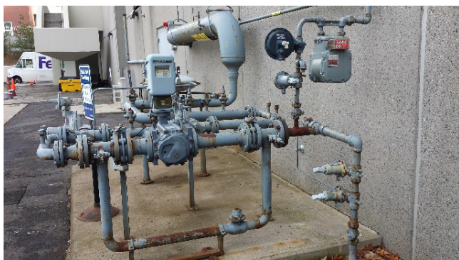
Existing Natural Gas Service at the SSC Building
